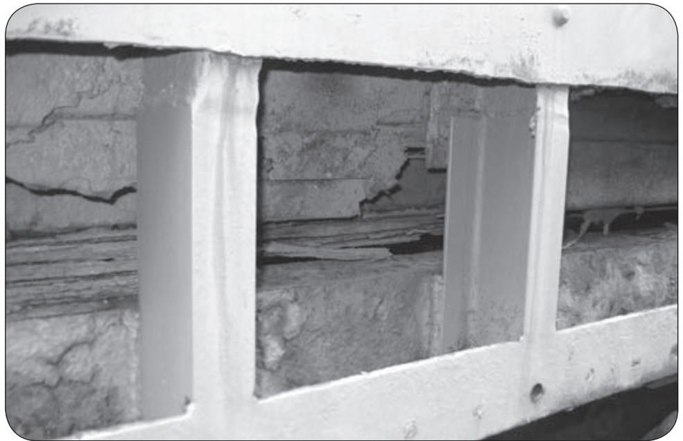
Old rusted vertical I-beams have been removed, and new beams have been welded in place for the side sheets. Midwest will cover this area with new sheet metal. (Photo by Michael Steinberg)
