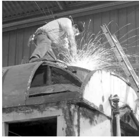
**Above: A Midwest employee welds the new sheet metal roof to the end of the 741. Note the visible curved support member. (Mike Steinberg photo)**
