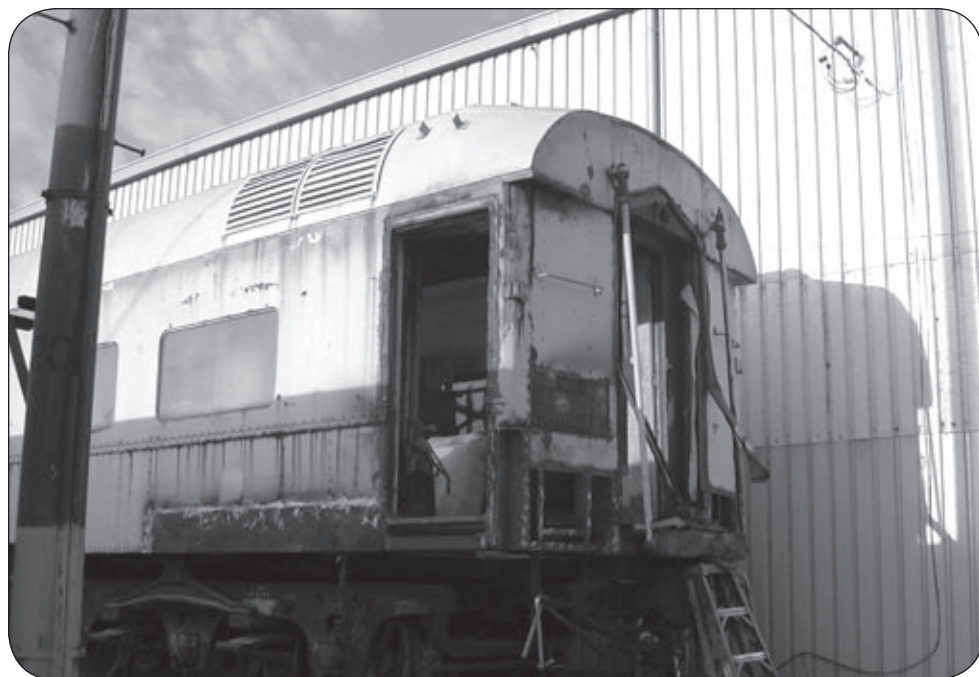
Diner 741 at Midwest Locomotive before metal work was completed on lounge-end.
